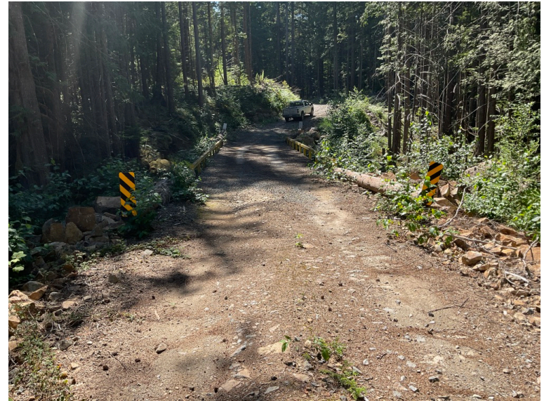
Approach from Right Bank when facing downstream
