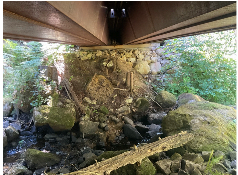
Left Bank Abutment when facing downstream
