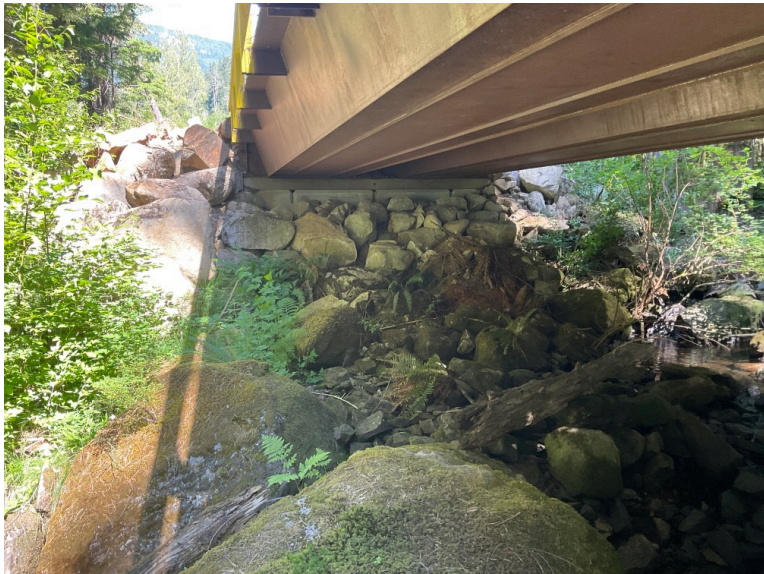
Right Bank Abutment when facing downstream
